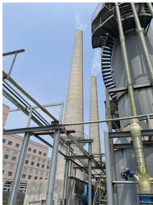
5#热媒站排气筒
